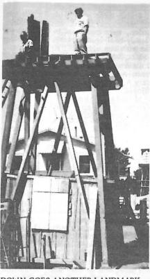
DOWN GOES ANOTHER LANDMARK This sturdy tower that once upheld a stout redwood tank for well water used on the site where Alpine Cottages are now, is being wrecked, as they hooked onto Rio SD MWD, so the tank is obsolete.
